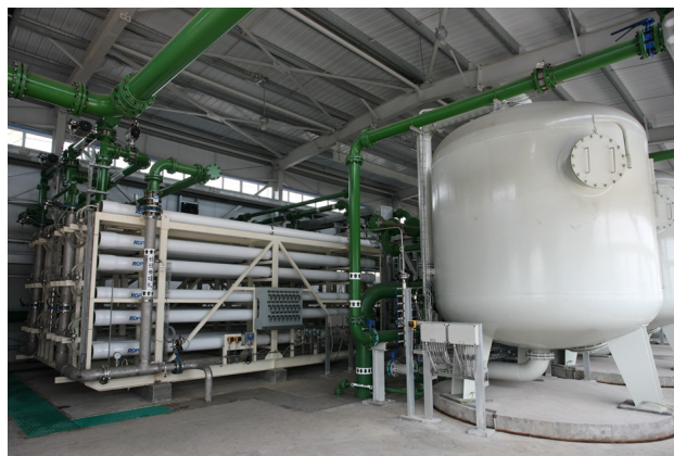
Part of the clean wastewater reuse unit
